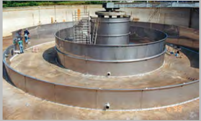
Edelstahlbehälter „Ring in Ring-System“ Stainless steel tank "System ring-in-ring"
