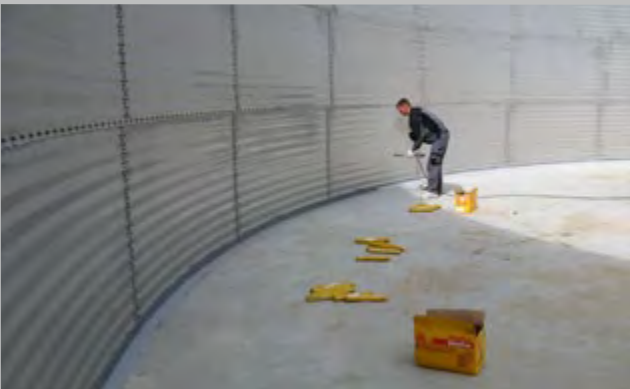
Wellstahlbehälter Montage innen Corrugated tank inside installation
