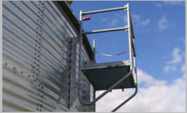
Arbeitsbühne am Edelstahlbehälter Working platform at stainless steel tank
